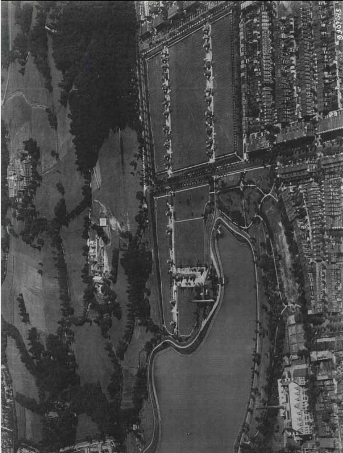
D-1: View of McMillan Sand Filtration Plant, looking north, Bolling Field Photo, Negative 9907 A.S. (summer 1921) RG 18AA, Box 153, No. 24 Courtesy of the National Archives Records Administration, Still Pictures Division
