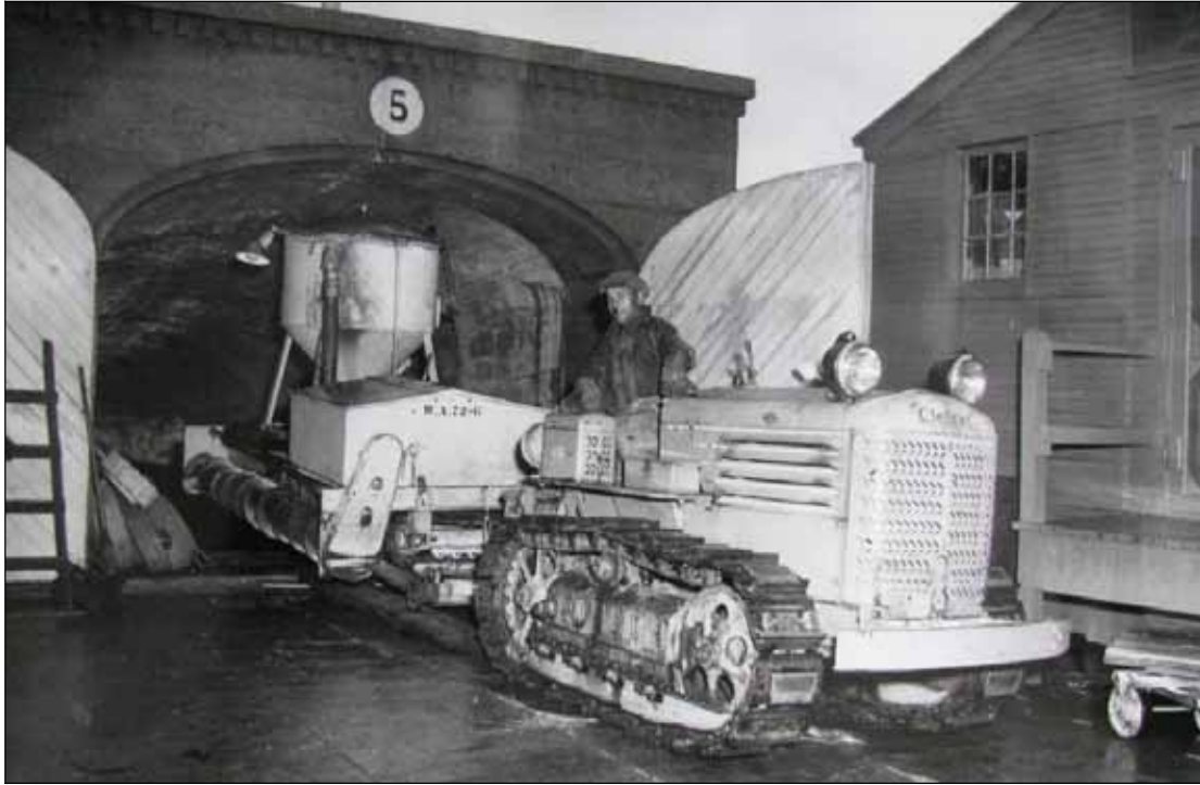
C-22: View of sand washing machine (c. 1944) Courtesy of the Archives of the Washington Aqueduct
