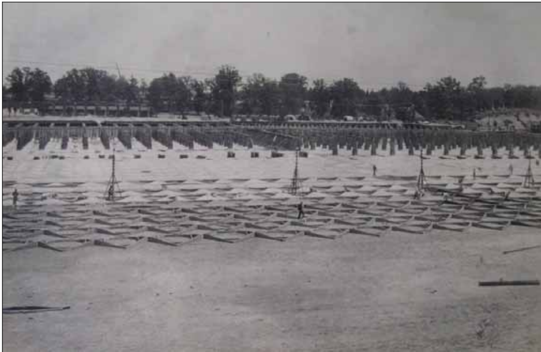
C-2: Concrete construction of filter beds (July 2, 1904) Courtesy of the Archives of the Washington Aqueduct
