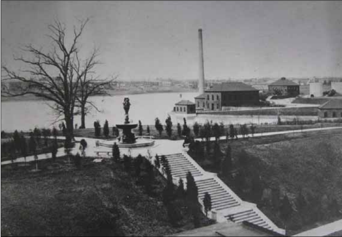
C-16: McMillan Memorial, east of First Street near intersection of Channing Street and First Street (c. 1911) Courtesy of the Archives of the Washington Aqueduct
