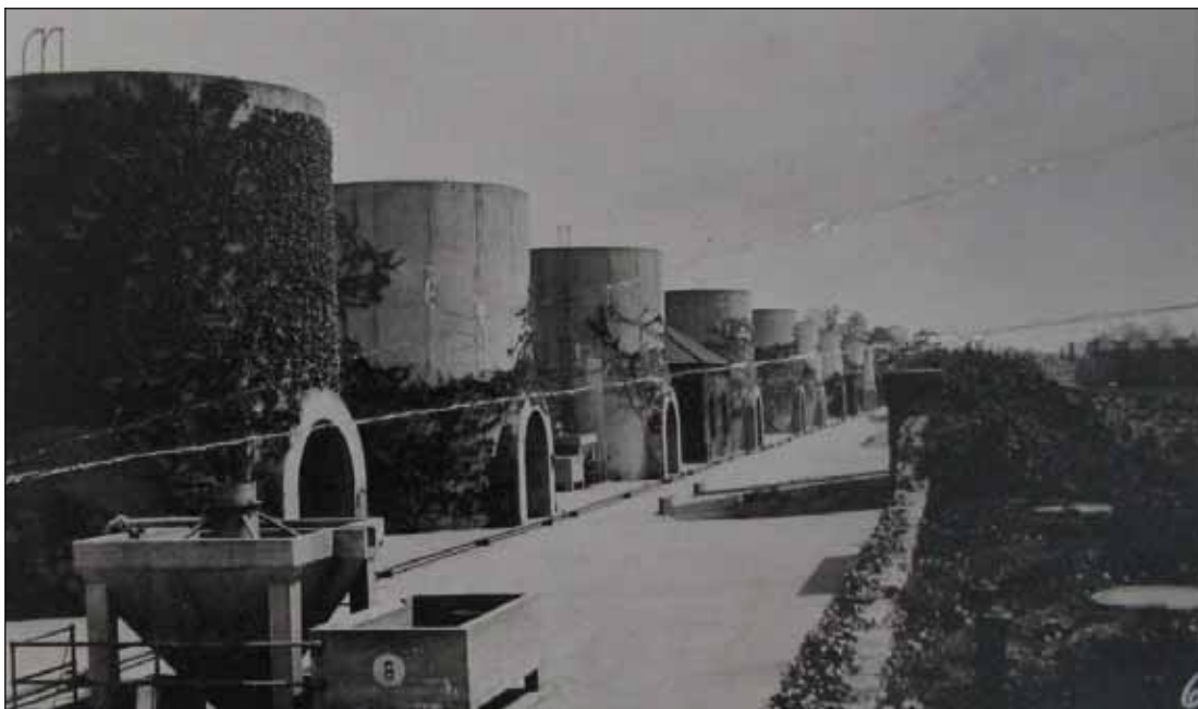
C-35: View of Court 2, looking east from First Street, NW (undated) Courtesy of the Archives of the Washington Aqueduct
