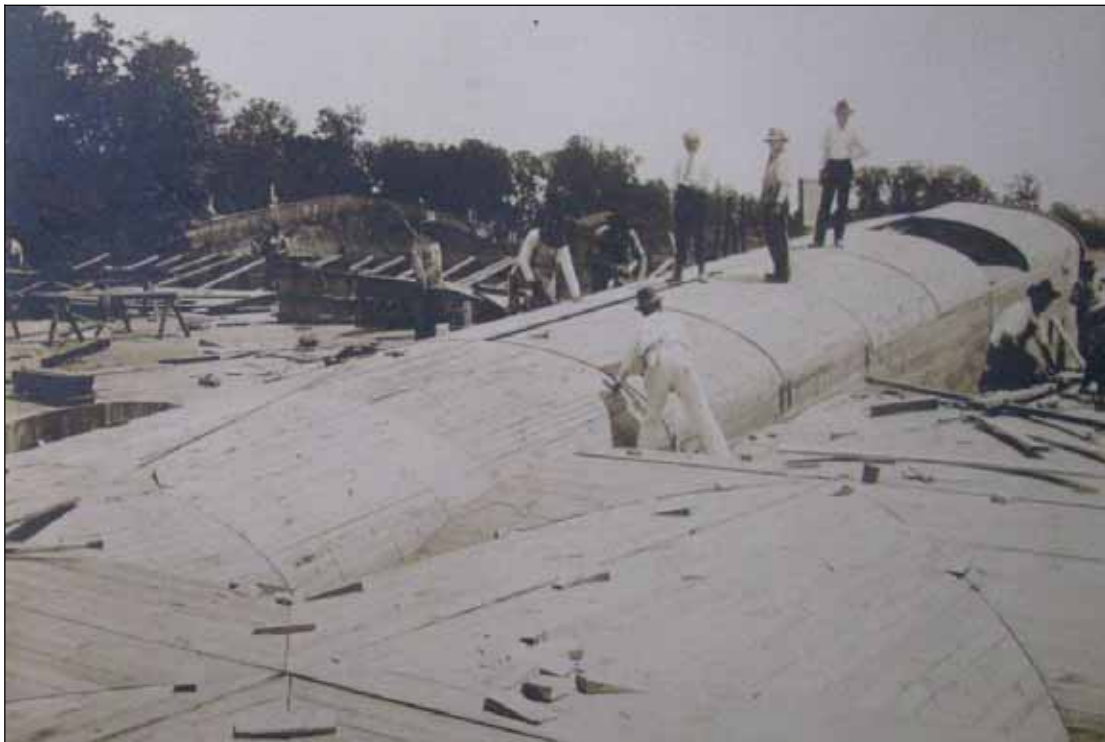
C-8: Form for entrance ramp to filter, looking northeast (1902-1904) Courtesy of the Archives of the Washington Aqueduct
