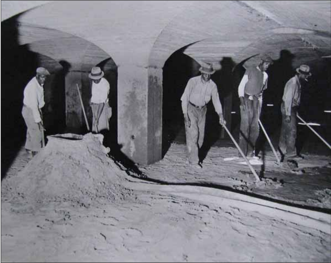
F-6: Workmen cleaning sand in filtration beds (c.1938) Washington Evening Star , from June 12, 1938 article Courtesy of the Martin Luther King, Jr., Memorial Library
