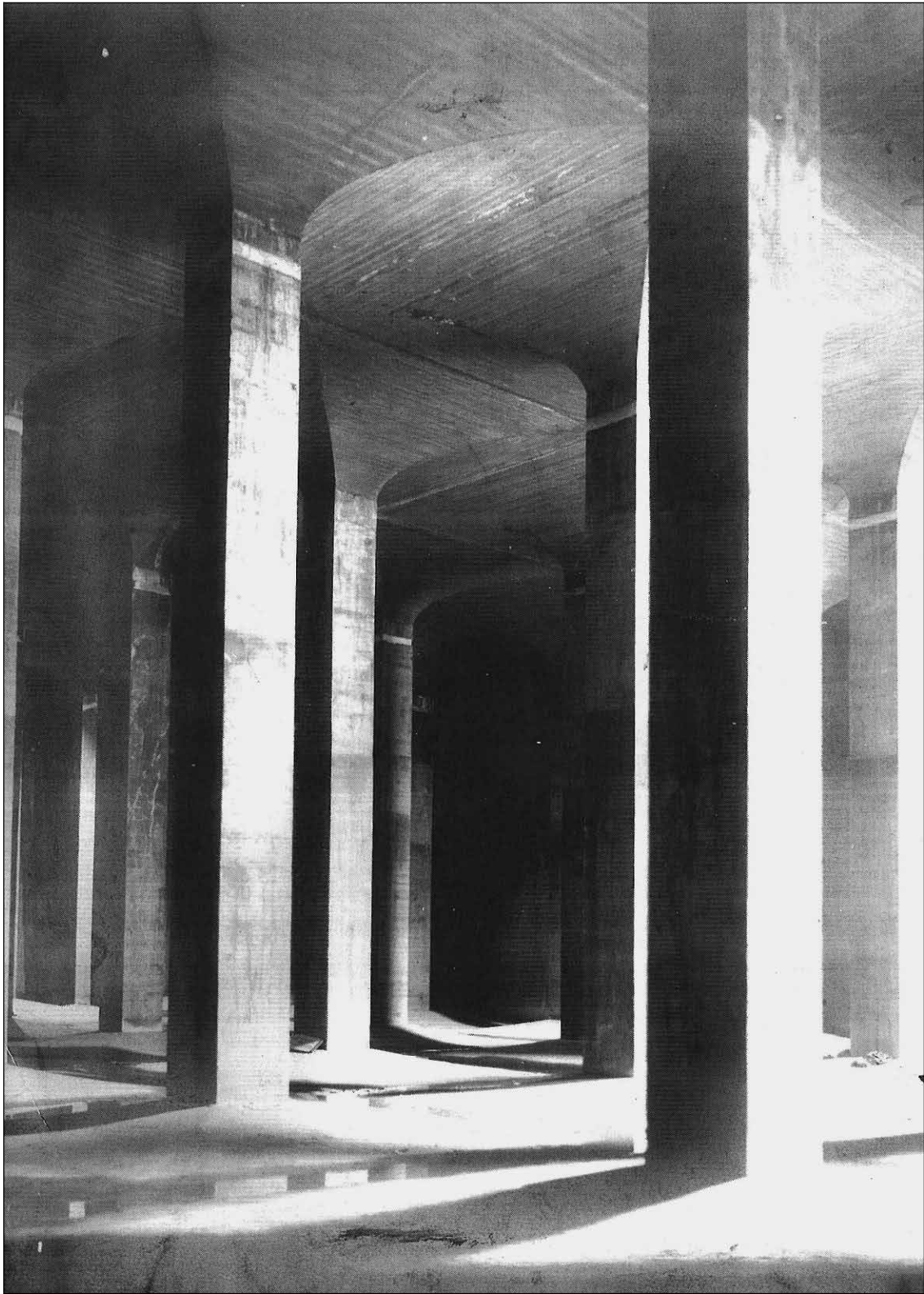
C-13: Interior view of north filtered-water reservoir (1902-1904) Courtesy of the Archives of the Washington Aqueduct
