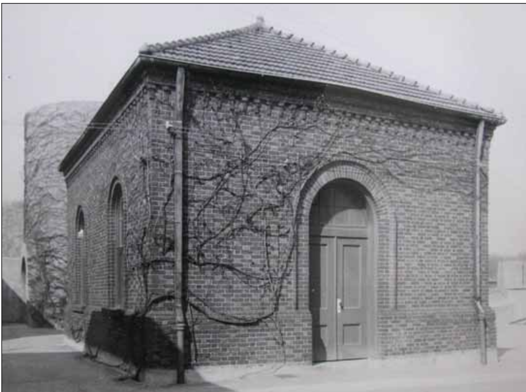
C-31: Regulator House 1, looking north (March 25, 1944) Courtesy of the Archives of the Washington Aqueduct
