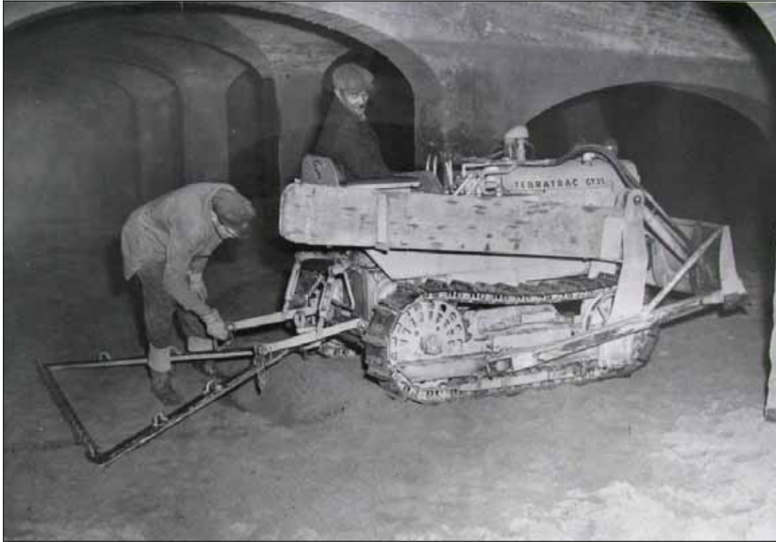
C-24: Tractor with filter rake (c. 1944) Courtesy of the Archives of the Washington Aqueduct
