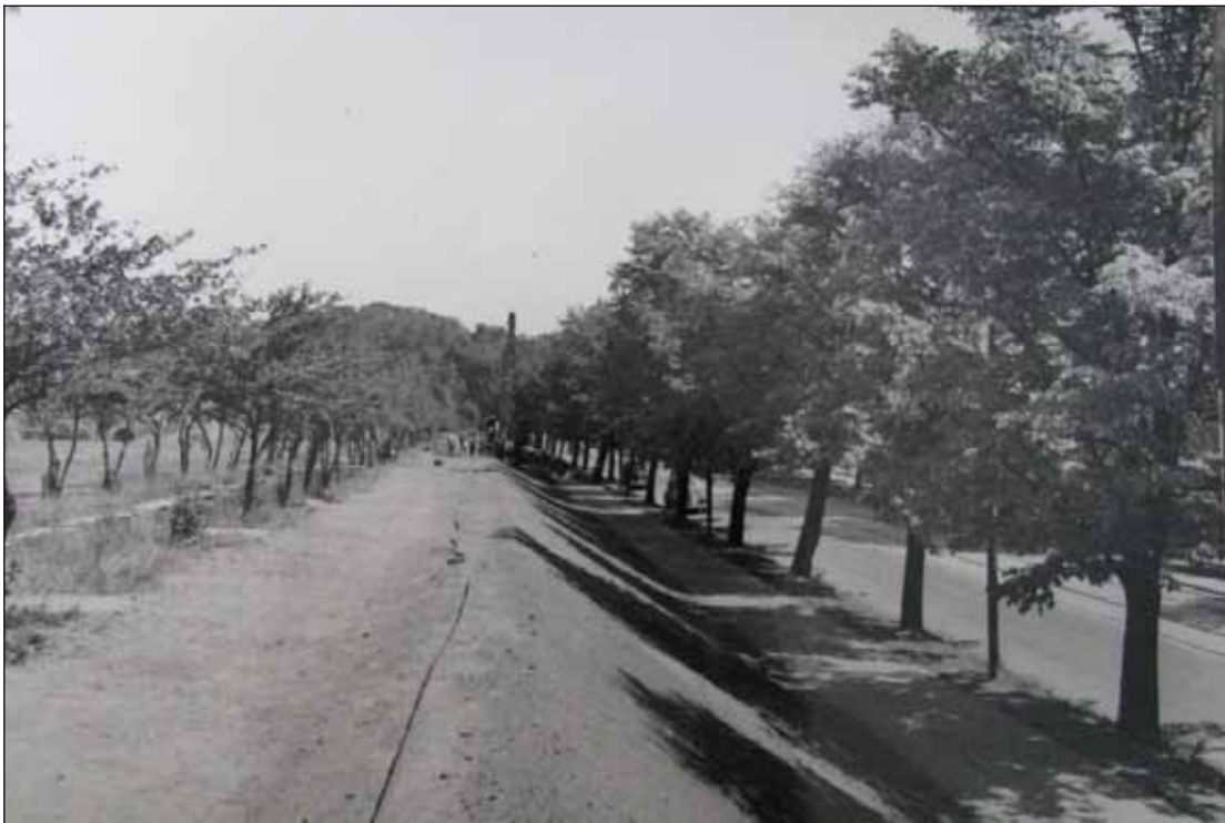
C-33: Construction of 36-in rising main loop, looking north on North Capitol Street from Court 2 (July 17, 1946) Courtesy of the Archives of the Washington Aqueduct
