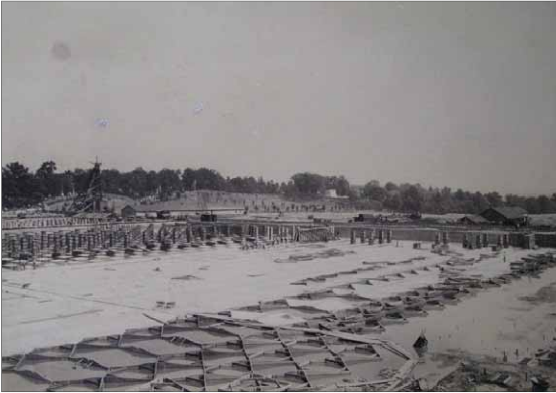
C-1: Concrete construction of filter beds (June 4, 1904) Courtesy of the Archives of the Washington Aqueduct
