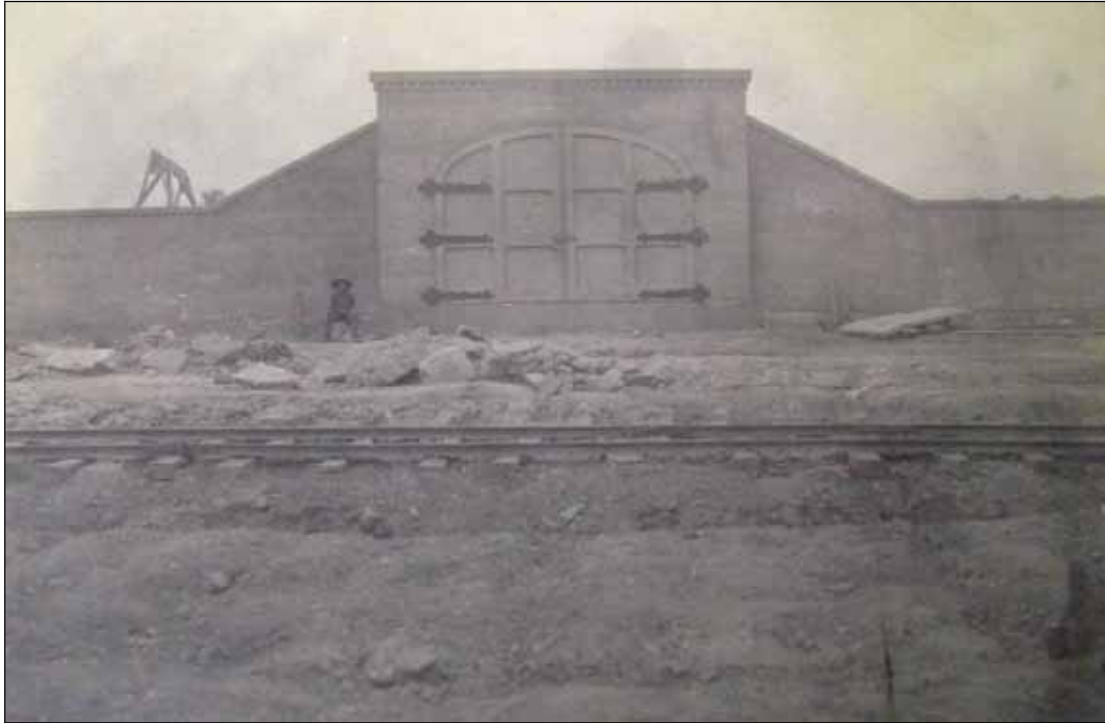
C-9: Door to filter bed (1902-1904) Courtesy of the Archives of the Washington Aqueduct
