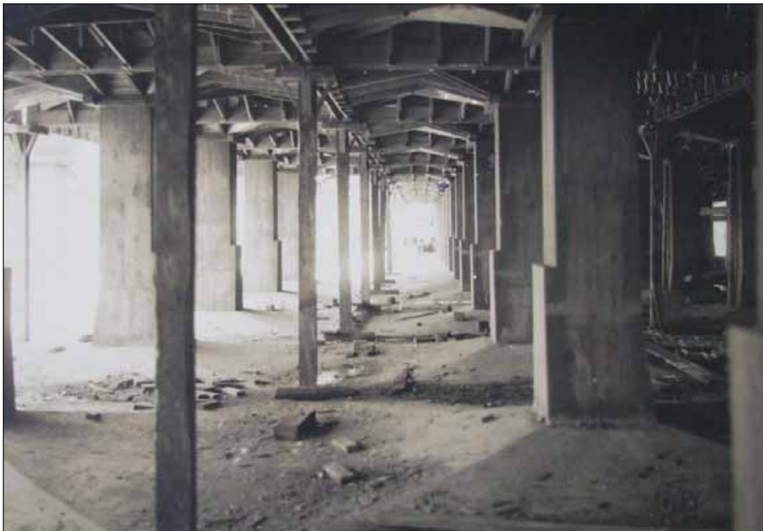
C-4: Centers for vaulting of filter beds (June 4, 1904) Courtesy of the Archives of the Washington Aqueduct
