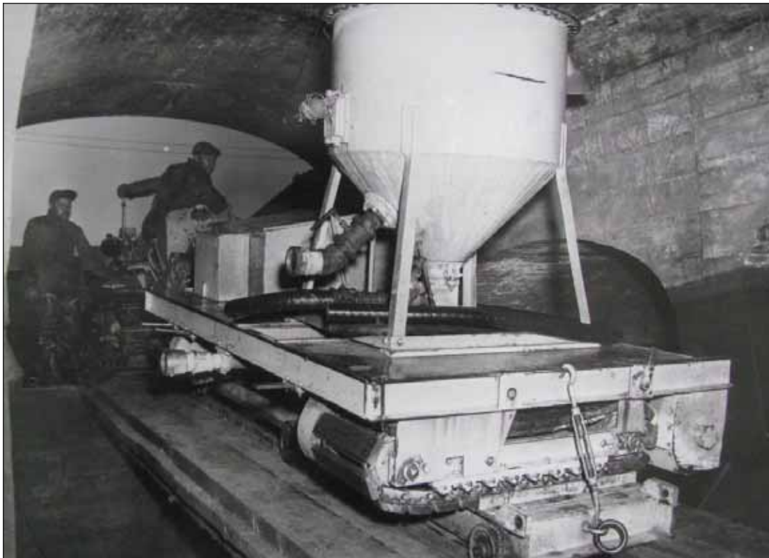
C-23: View of sand washing machine as carried on dolly down filter entrance ramp (c. 1944) Courtesy of the Archives of the Washington Aqueduct
