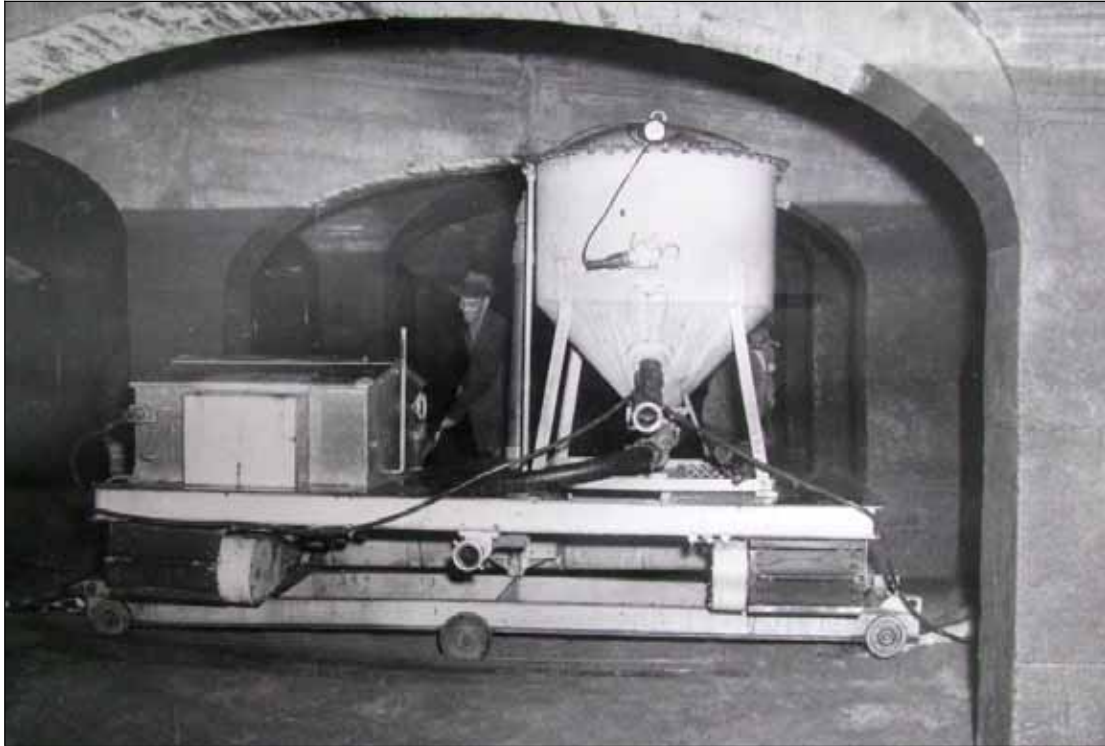
C-26: Transport of sand washing machine on dolly over metal channels (c. 1944) Courtesy of the Archives of the Washington Aqueduct
