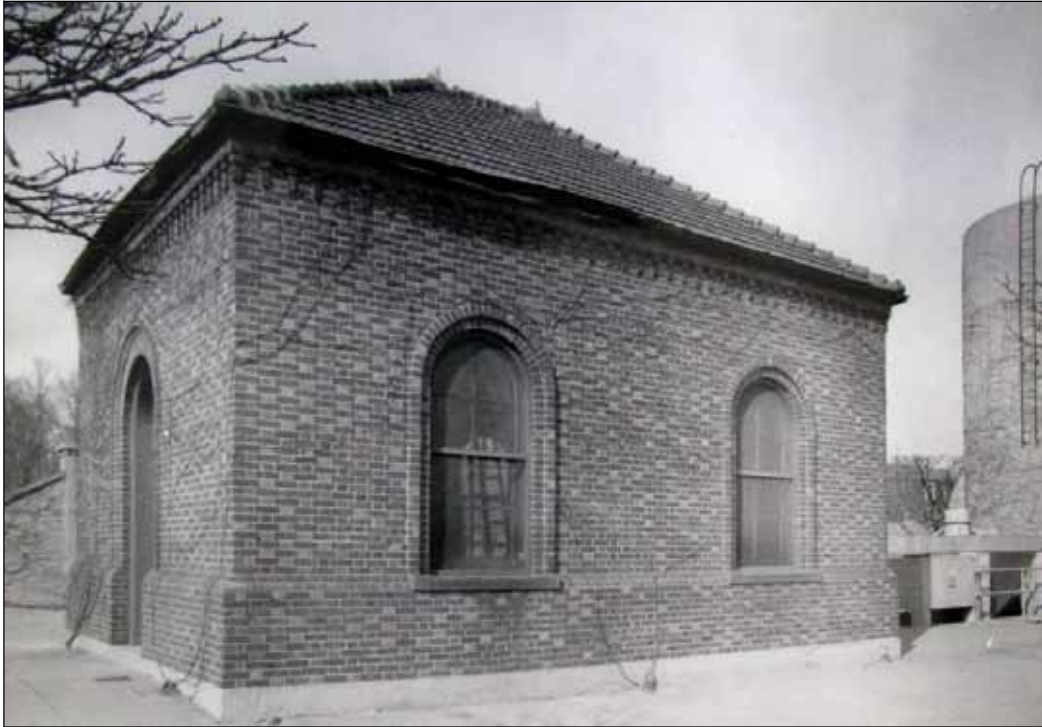
C-30: Regulator House 5, looking northeast (March 25, 1944) Courtesy of the Archives of the Washington Aqueduct
